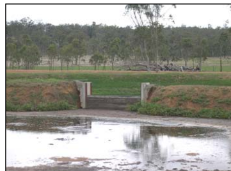
Settling basin with drop board weir
