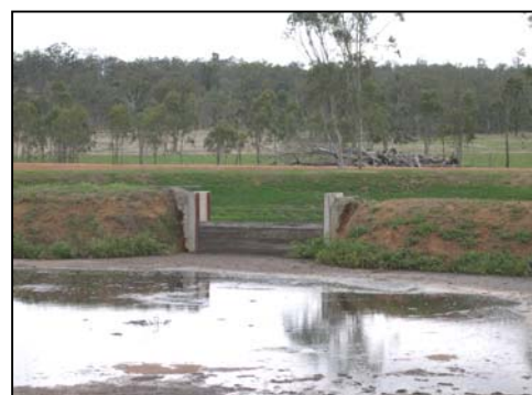
Settling basin with drop board weir
