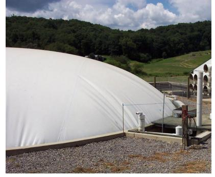
were, namely a Covered Anaerobic Lagoon or CAL or a Completely Stirred Tank Reactor or CSTR. Efficiency of the CSTR is generally superior to a CAL system, however the capital cost is high.
